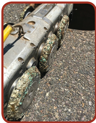
Figure 24: CCTV wheels show evidence of damage to flexible thermoplastic pipe.
