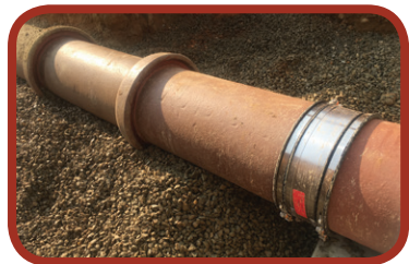
Figure 21: A finished repair coupling near a manhole.
