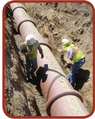
Figure 23: Shovel slicing the pipe haunches
