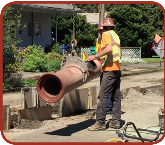
Figure 16: Repairing a length of pipe in an older, established community.
