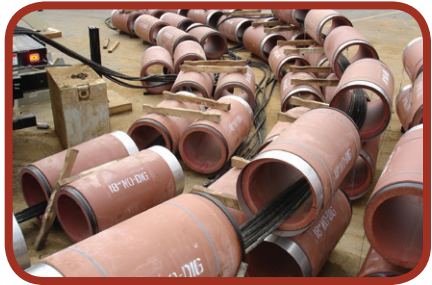
Figure 38: Jacking pipes staged at the launch pit on a pilot tube project utilizing a powered cutter head.
