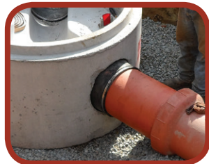
Figure 33: Two points of flexibility at this manhole are provided by the flexible manhole connector and the flexible compression joint on the short length of pipe.
