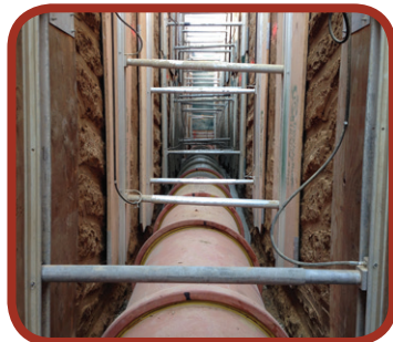
Figure 6: Trench sheeting and spreader bars
