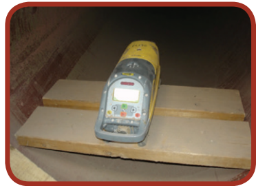
Figure 3: A common pipe laser in use
