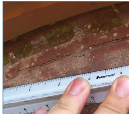
Figure 30: Crazing (pictured here) is common, but it has also been misidentified as a fracture or crack.
