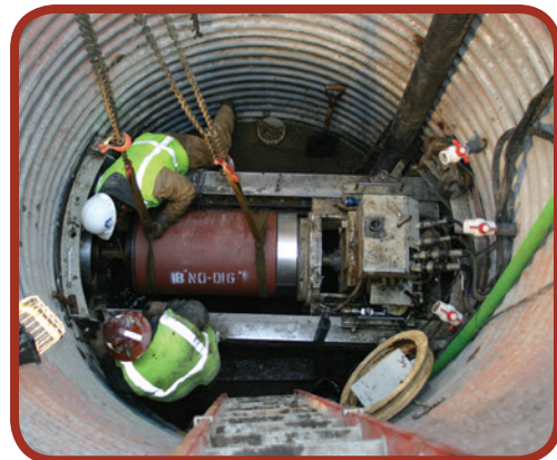
Figure 8-7: 8 Ft. round jacking shaft and pilot tube frame.
