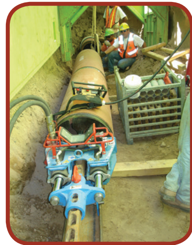
Figure 8-18: Launch pit showing cylinder pack, bursting rods, pipe sections, and expander.
