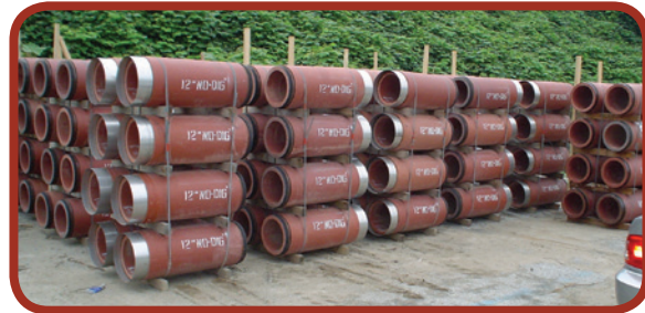
Figure 8-4: Jacking pipe utilize a series 316 stainless steel collar at each compression joint.
