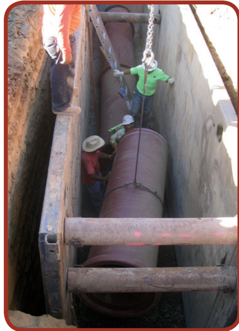
Figure 7-4: Trench Box within the pipe zone
