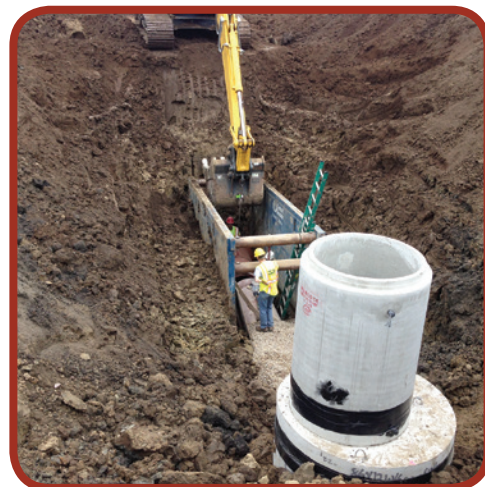
Figure 7-15: Pulling a trench box within the limits of the pipe zone.
