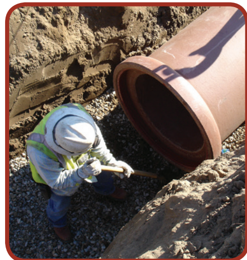
Figure 7-5: Constructing a bell hole during pipe laying
