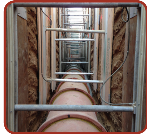
Figure 7-2: Trench sheeting and spreader bars
