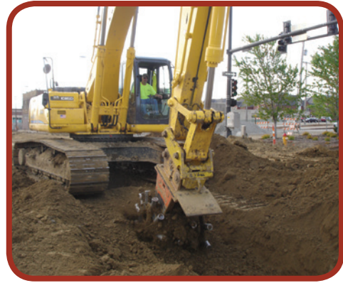
Figure 7-11: Hoe mounted sheepfoot roller compacting final backfill
