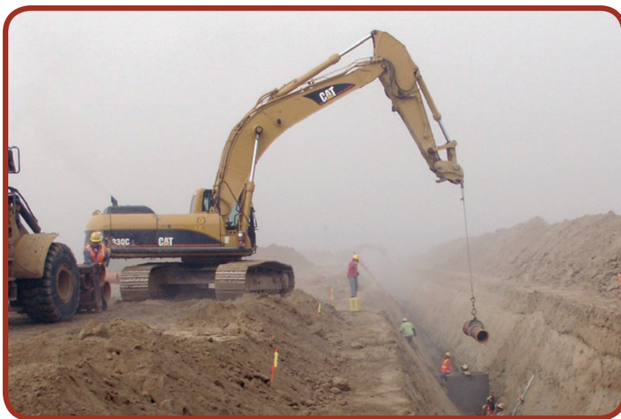
Figure 7-1: Open trench construction utilizing a modified vee trench.
