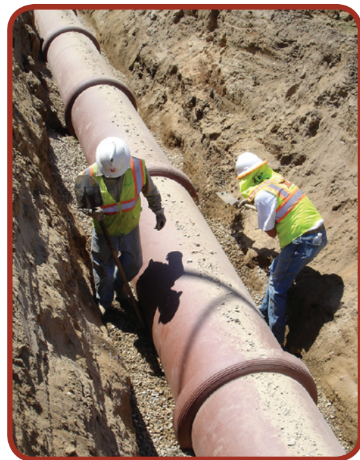
Figure 7-10: Shovel slicing the pipe haunches
