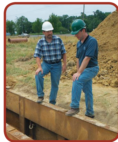
Figure 11-3: Inspectors are a vital link between specification and construction.
