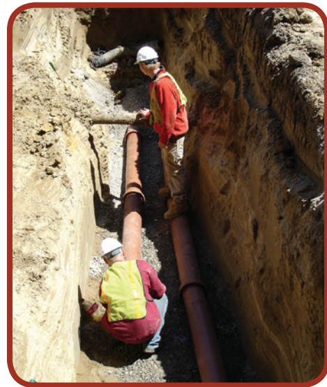
Figure 10-3: Two services constructed in the same trench excavation.
