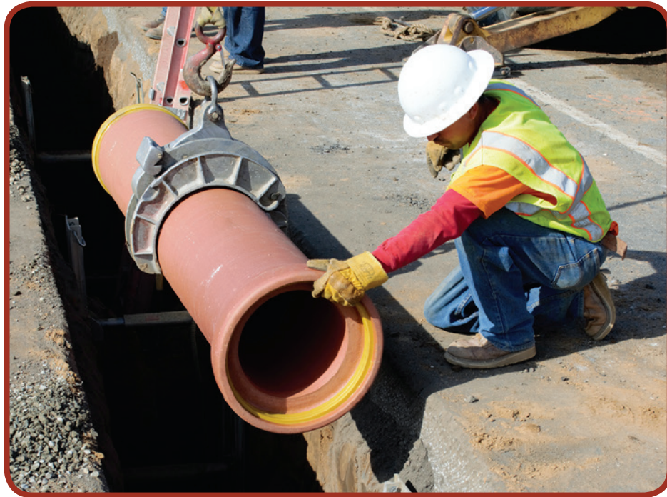
Figure 1-1: Modern Vitrified Clay Pipe (VCP) with factory-applied, compression joints, which “shall not leak,” per ASTM C425.
