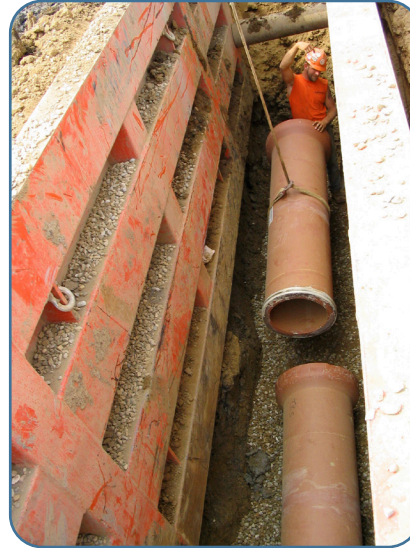
Figure 11: Open Trench Installation
