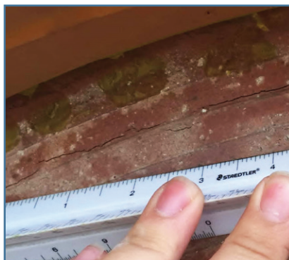
Figure 30: Crazing (pictured here) is common, but it has also been misidentified as a fracture or crack.
