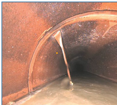
Figure 29: CCTV image of polyurethane gasket overpour
